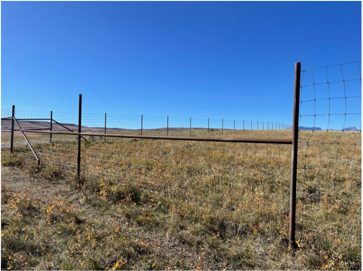
Field fence folded over as overpass:
